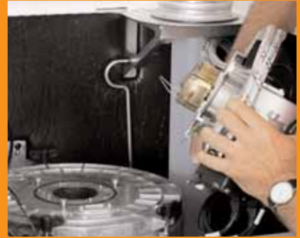
Take out the burner unit
