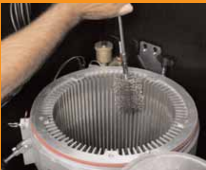
Brush the heat exchanger clean
