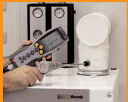
Install the housing and check the combustion parameters
