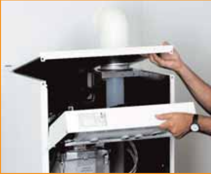
Open the housing and open the bottom-hinged controller box
